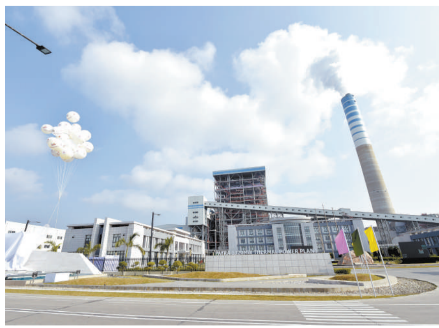
The 1.32 GW ultra-supercritical coal-fired power plant in Patuakhali, Bangladesh. (PHOTO: XINHUA)
